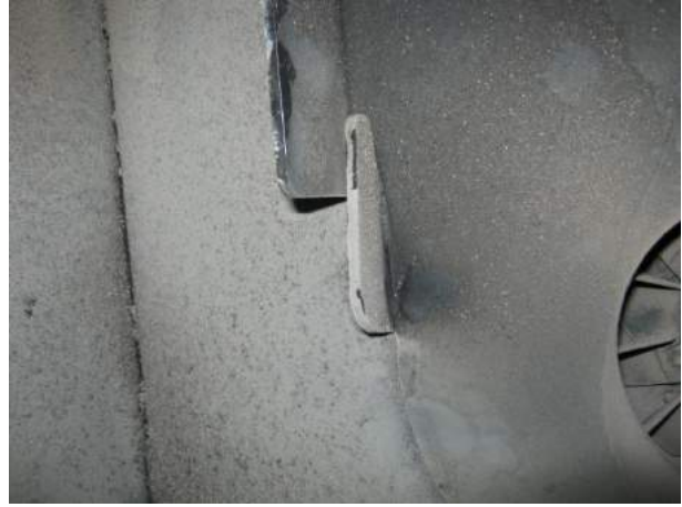
Combustion Air Cover Repaired Position for Run 2
