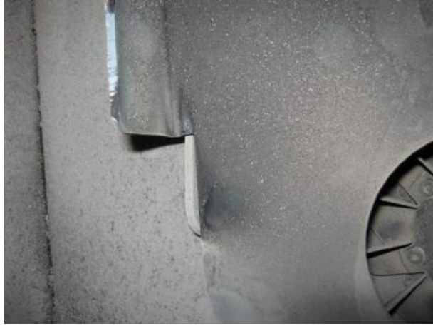
Combustion Air Cover As Received Position for Run 1
